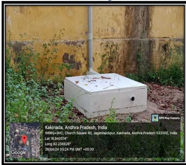
Ground Water Recharge Pits 2
