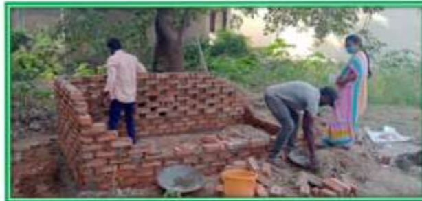
NADEP Compost Pit work started on 05.03.2022. Principal Dr.V.Anathu Lakshmi Madam monitoring the construction of the Compost Pit.
