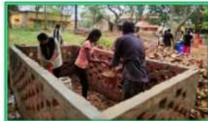
Planting the of NADEP Compost Pit walls with Cow dung by students.
