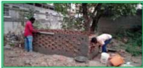
Construction of the NADEP Compost Pit completed.
