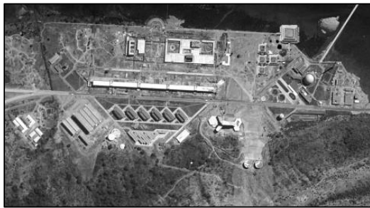
Apsara reactor - Asia's first nuclear reactor. 1 MW, pool type, light water moderated, highly enriched (93%) uranium fuel supplied by France
